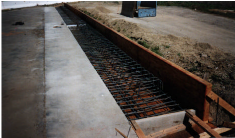
Figure 2-2 - Concrete Anchor Block with Simulated Bridge Deck Reinforcing Steel
