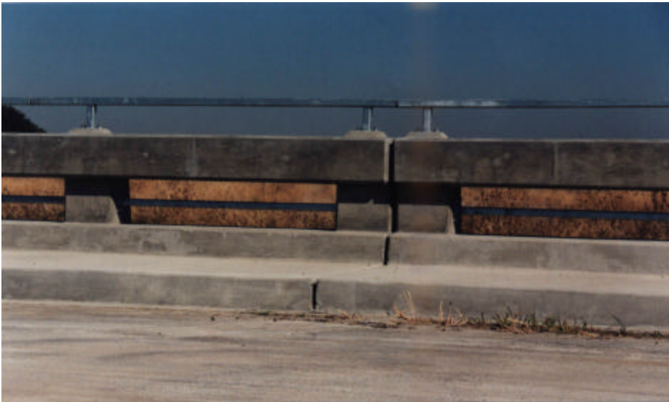
Figure 2-12 - Completed Expansion Joint
