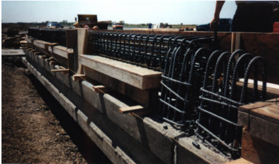
Figure 2-8 - Expansion Joint Post and Beam Configuration
