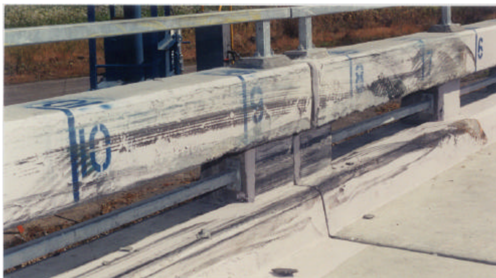
Figure 2-41 - Impact Area and Expansion Joint
