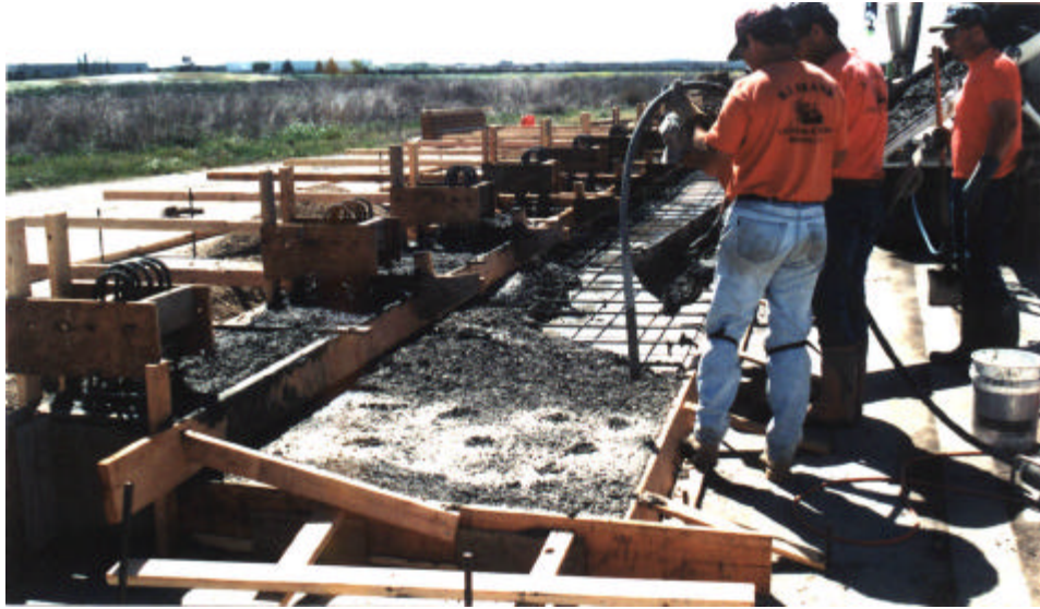
Figure 2-5 - Concrete Pour for Sidewalk and Curb Section of Bridge Rail
