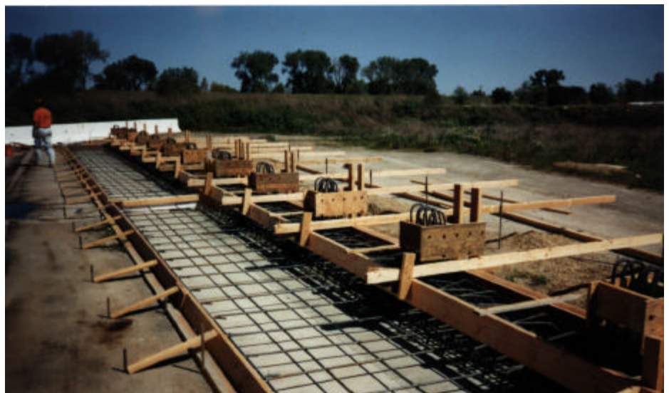
Figure 2-4 - Reinforcing Steel for the Sidewalk and Lower Portion of the Bridge Rail
