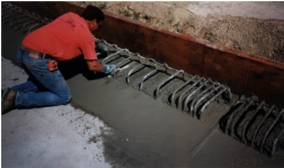
Figure 2-3 - Simulated Bridge Deck Construction
